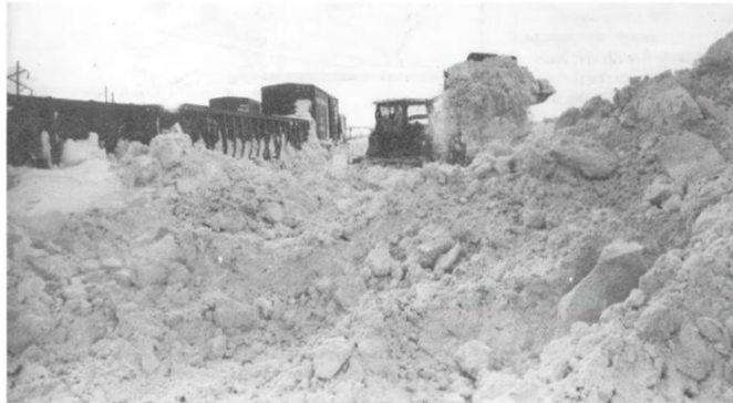
CLEANING UP the yards were front end loaders that worked in restricted areas where plows couldn't function.
