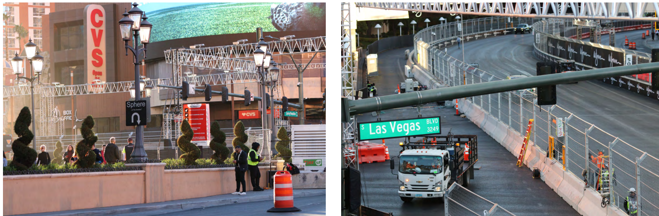
Figure 32. Formula One Grand Prix construction Credit: RTC Southern Nevada
