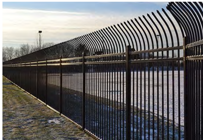
Figure 35. Security fencing Credit: MBTA
