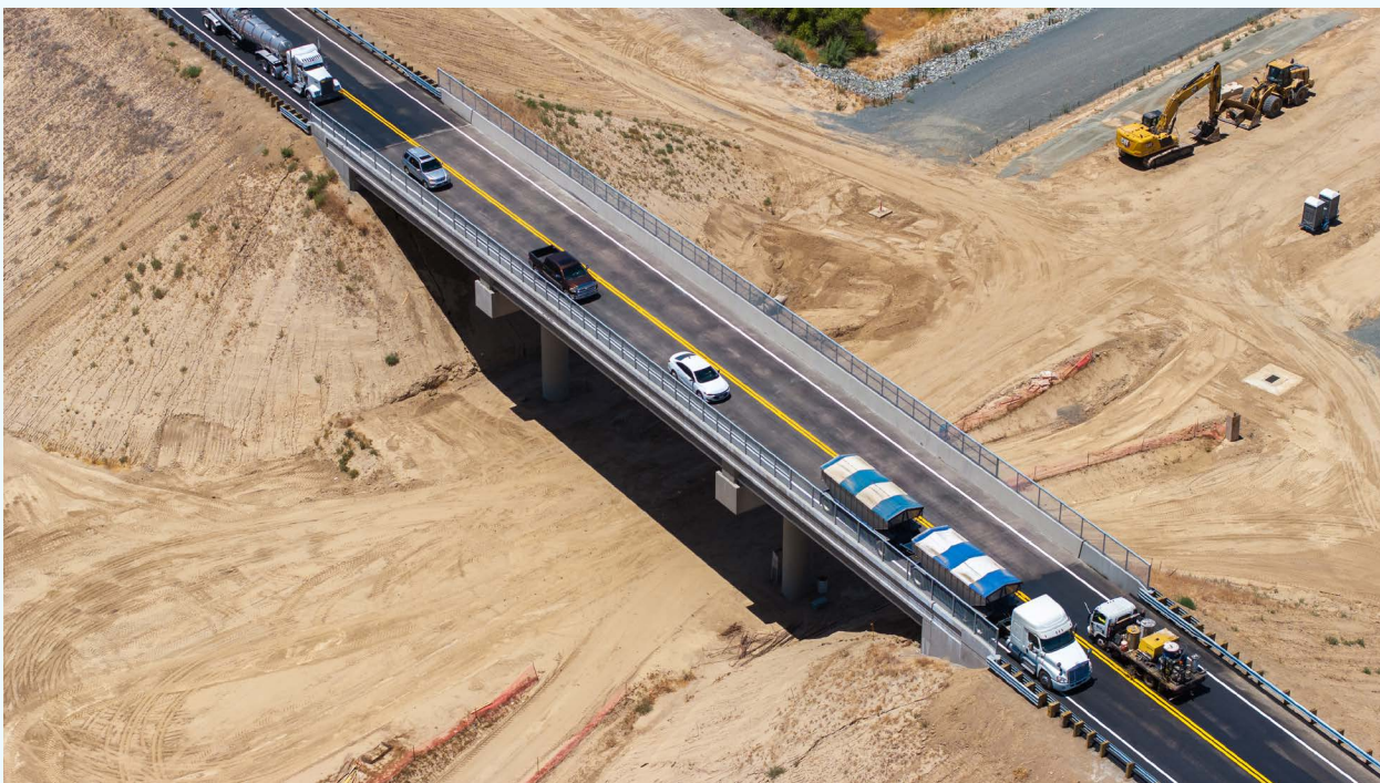
The Avenue 56 Grade Separation in Tulare County was completed in June 2025 and spans a length of 219 feet.
