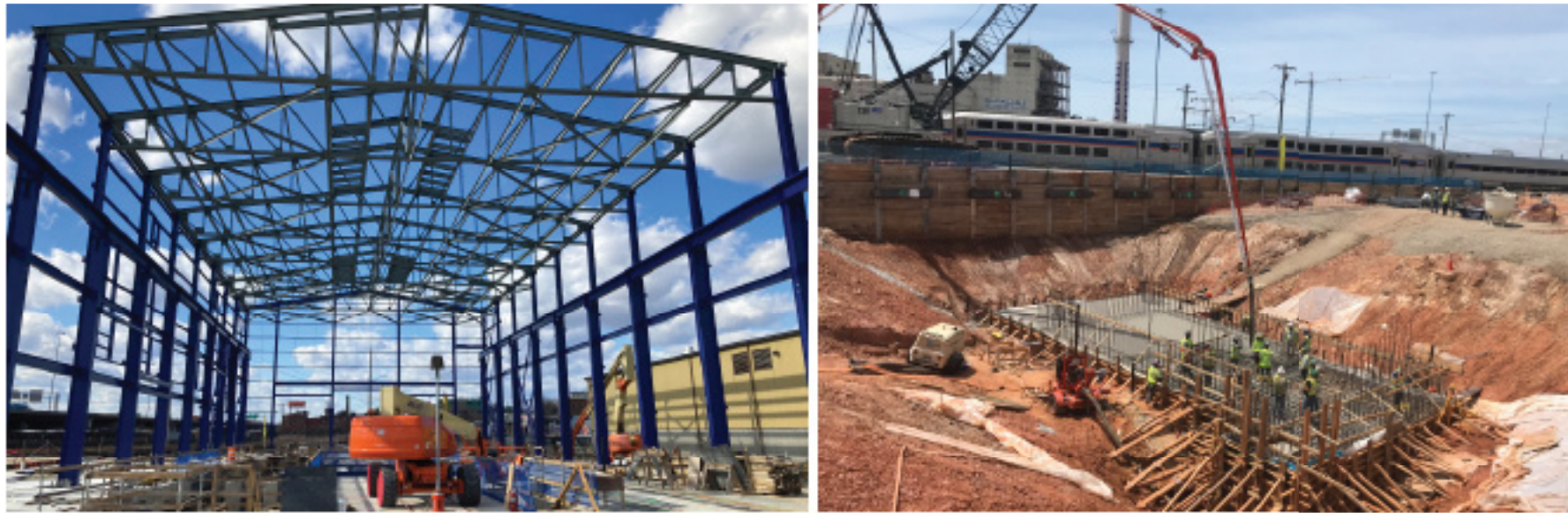
New Marc Train Riverside Heavy Maintenance Building
