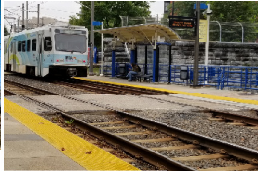
Light Rail Catenary System Rehabilitation
