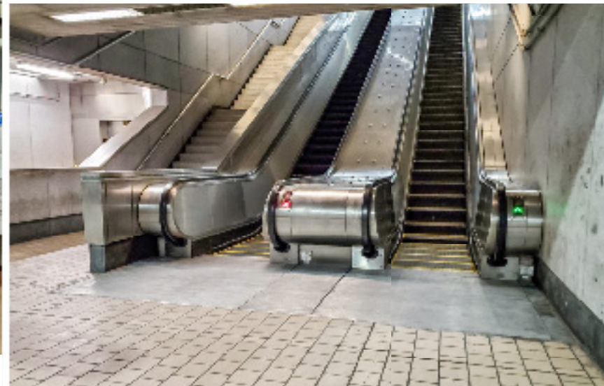
Penn-North Escalator Replacement
