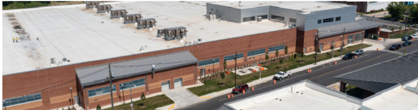
Kirk Bus Division Modernization Phase 2
