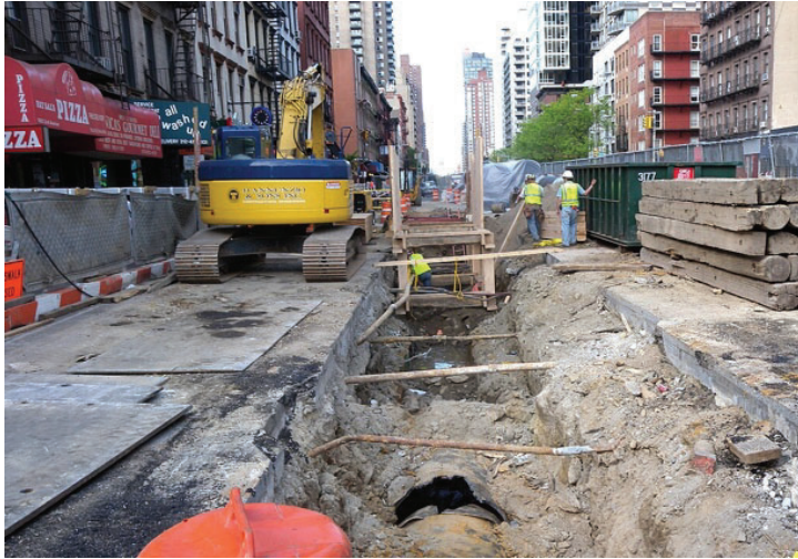
Construction required replacing numerous utility lines. Source: Wikipedia .
