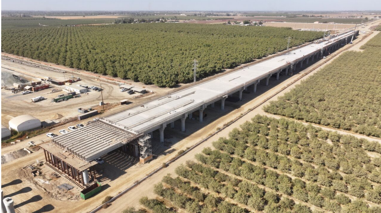
The Hanford Viaduct in Kings, California
