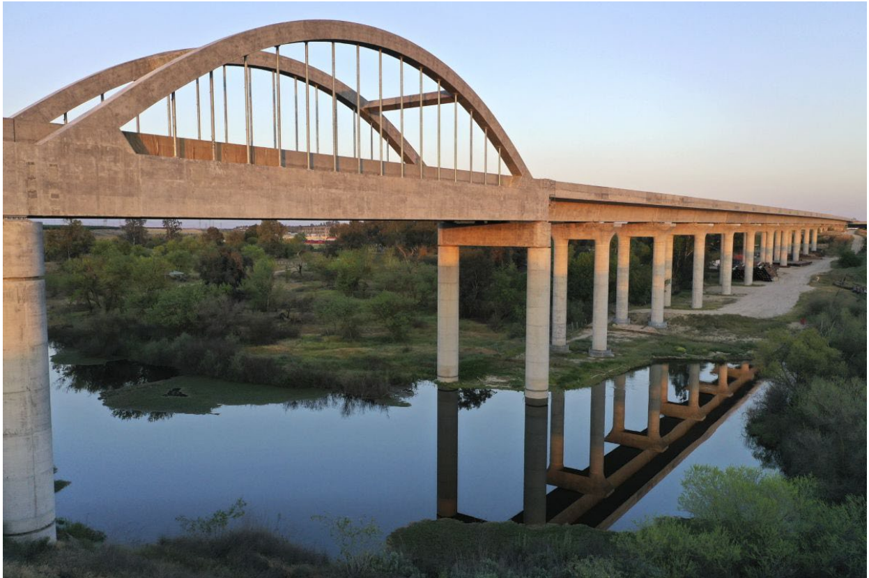
The San Joaquin River Viaduct in Fresno, California
