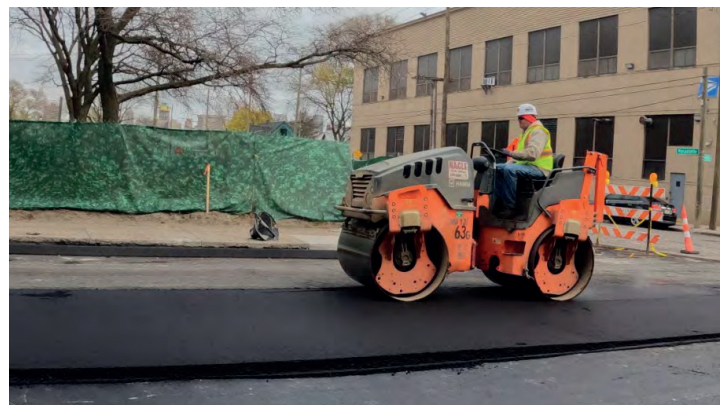
Roller compacting new pavement on 14th Street
