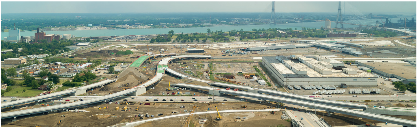
GHIB U.S. Port of Entry Progress
