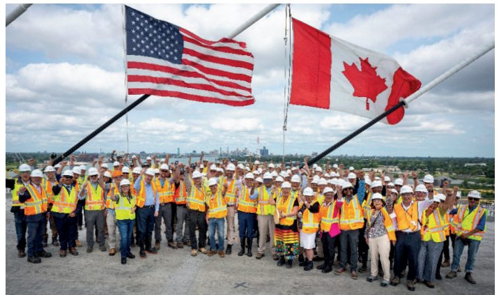
Workers, officials and the family of Gordie Howe celebrate the joining of the bridge deck in July 2024
