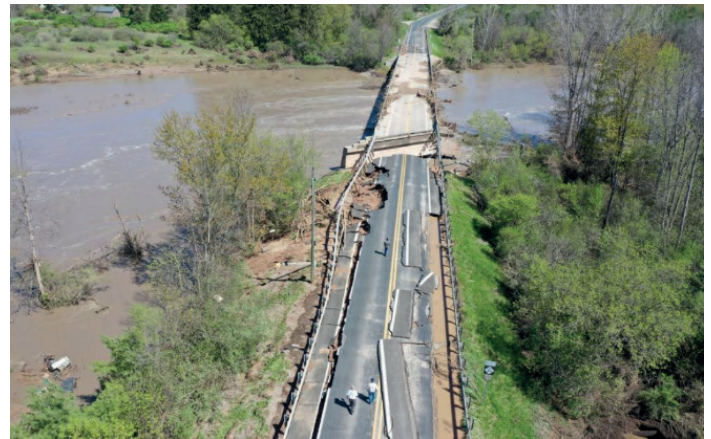
Roadway flooding and damage in Midland County
