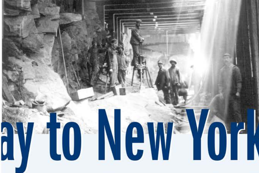
Far left: Building is under way on the Lexington Avenue Line south of City Hall Station. (Park Row; 1902)
