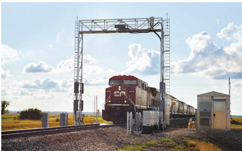
CP's Train Inspection Portal System
